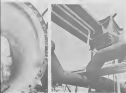
Welders G. Tromp and M. Lopez (r) join two pipe lengths in Welding Shop to make 80 ft. long sections.
